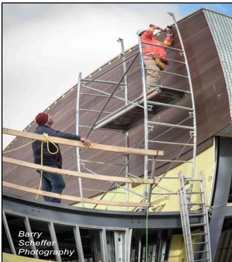
Workers adding wood siding to the raised section of the banquet hall roof.
